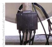
We need to think about where we are going to place the DiSEqC switch. In most cases the box is attached to the pole behind the dish. The reason we have to know the location at this stage
